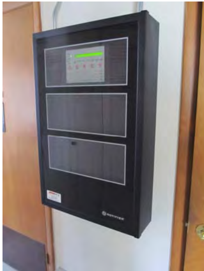
Newer, fully addressable, fire alarm control panel located at community building – Panel also reports to panel located at adjacent Orchard Hill Estates I development
