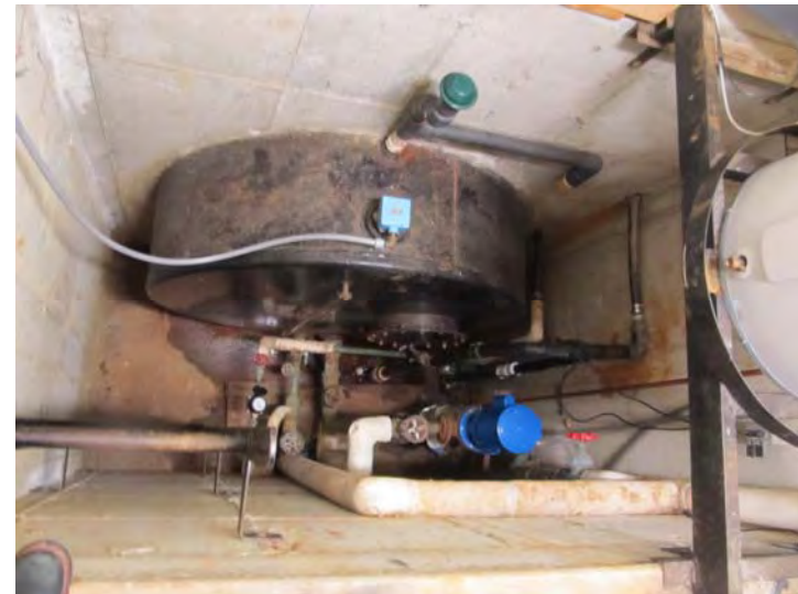
Nose view of underground steel storage tank and pressure pump (in blue) components of well water system that serves development
