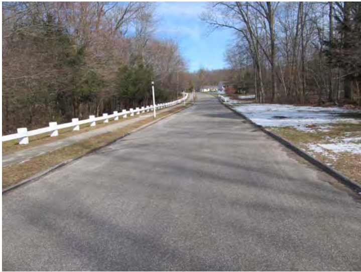
Asphalt-paved access drive with wood guard rail and typical site lighting fixture
