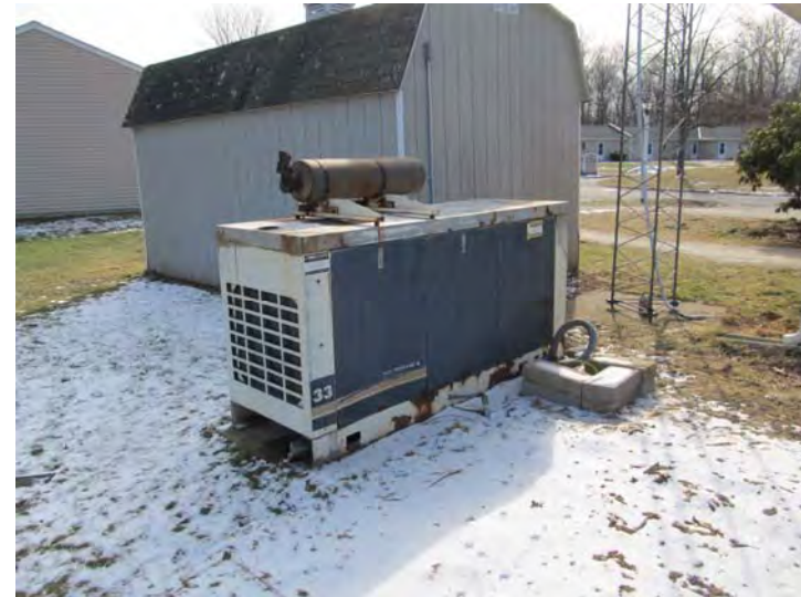
Original propane-fired emergency generator that serves community building and well water system
