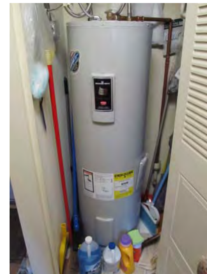
Each unit has an electric, storage-type, domestic hot water tank – All recently replaced
