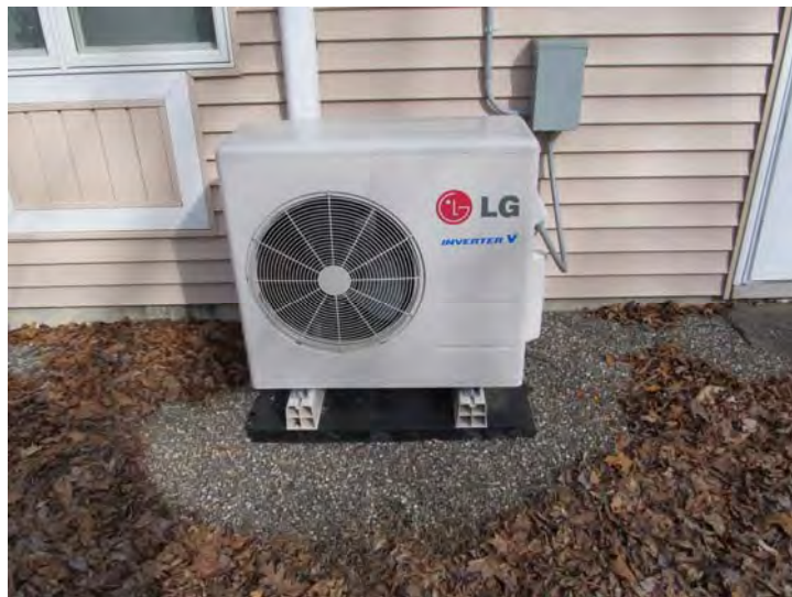
Typical exterior, air-cooled, condenser for heat pump systems recently installed at all units
