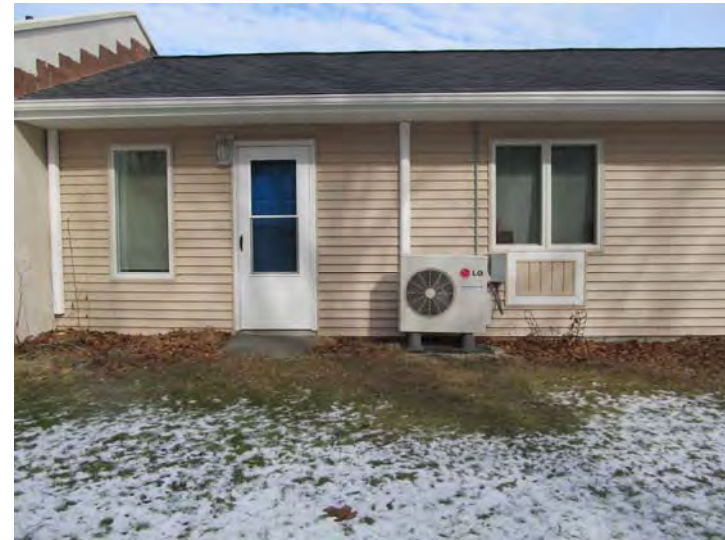
Renovation work completed during 2011 included new vinyl siding, windows, and storm doors – All components in good overall condition at the present time
